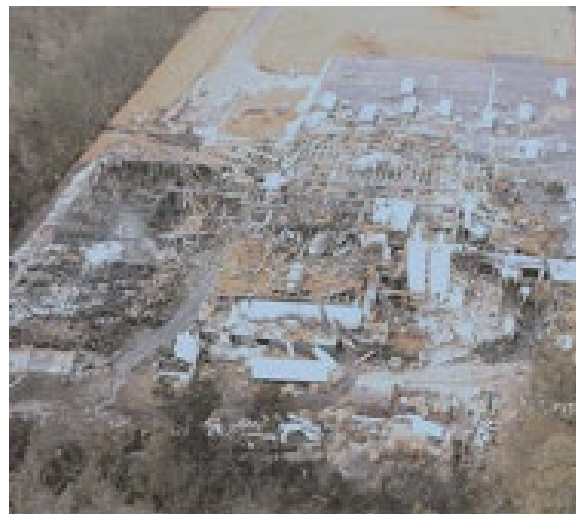
A pharmaceutical plant after a dust explosion.
